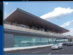
DULLES CORRIDOR METRORAIL
