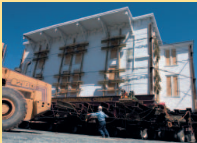
Placed on wheels, Varsity Hall was rolled 185 feet down an eight-degree slope of packed gravel to its new location on Hospital Drive.
