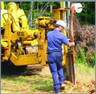
Cable plow installing fiber optic cable.
