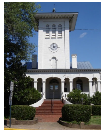
Orange County Courthouse
