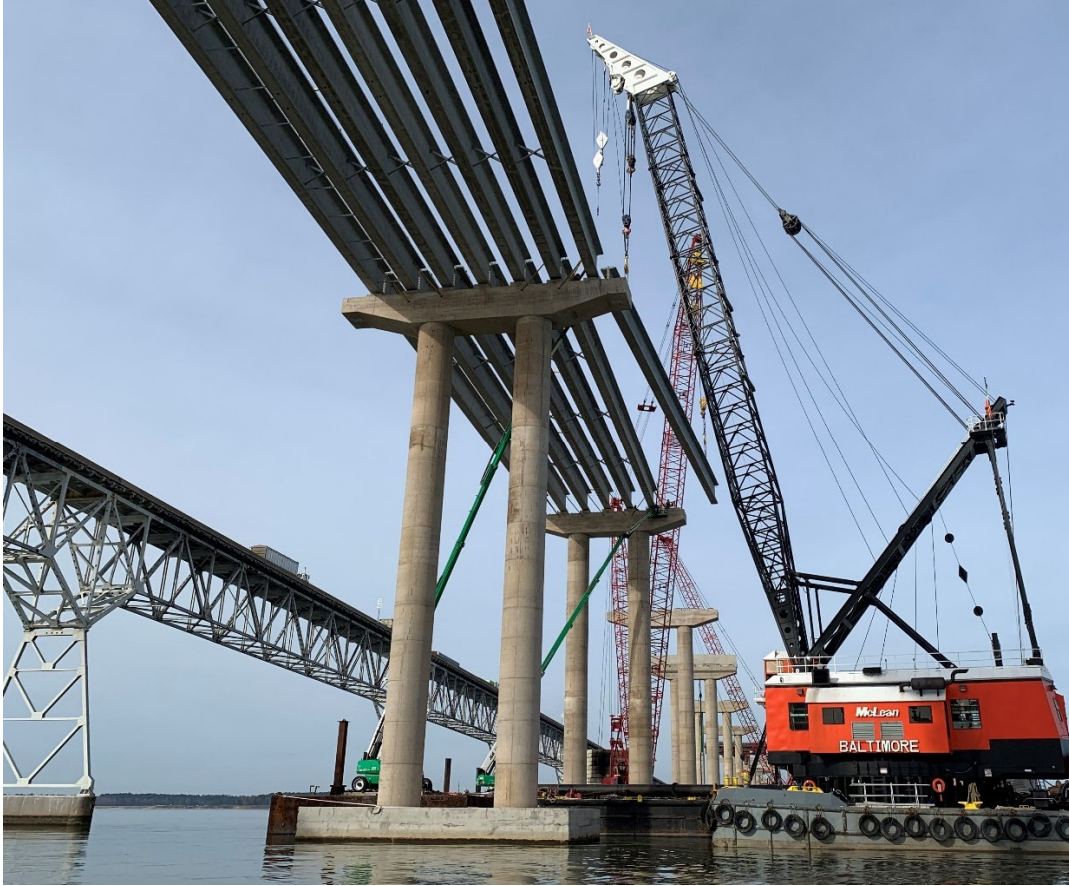
Harry Nice Bridge – Crossing Potomac River - manufactured in Cape Charles at Coastal Precast
