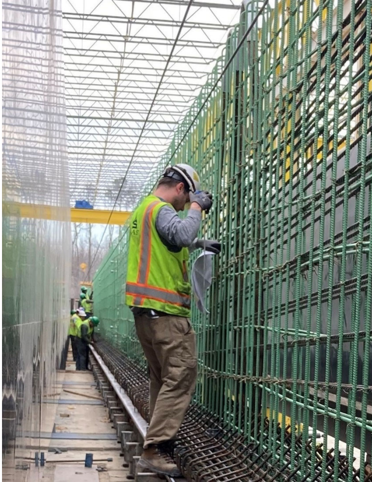
Employees tie steel for Harry Nice Bridge Beams at Coastal Precast in Cape Charles
